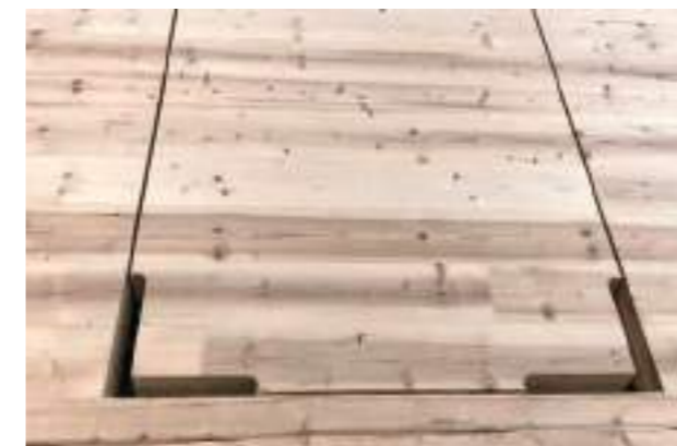
Cut-out, residual radii removed
