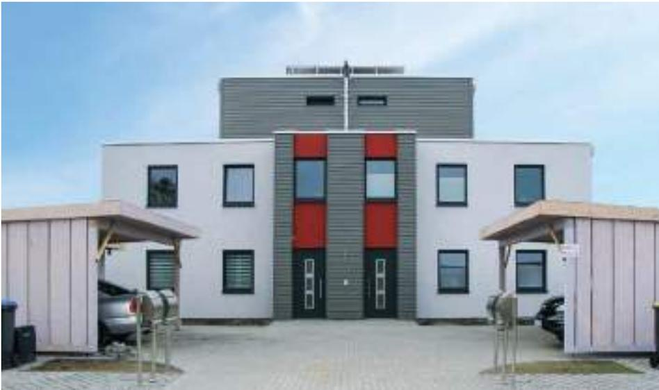
In this 3-storey building with 400 m<sup>2</sup> living space for a total of four families, the outer and inner walls as well as the ceilings and the roof consist of **MMHBE** elements.
